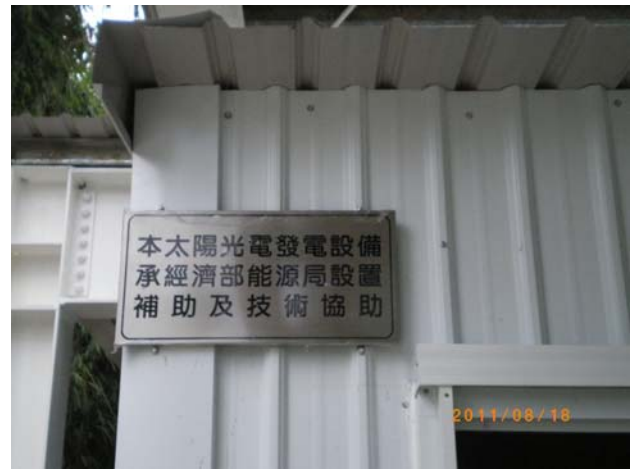
The brand named solar energy equipment has a total capacity
